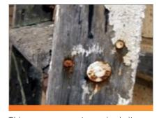
This rung was not repaired, it was made even more unsafe! It is kept "firm" by nails which are already badly corroded.
